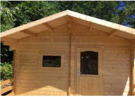
41. View of sauna after fascia boards attached.
