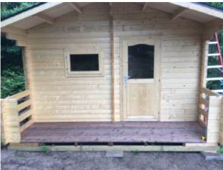
43. View of completed porch.
