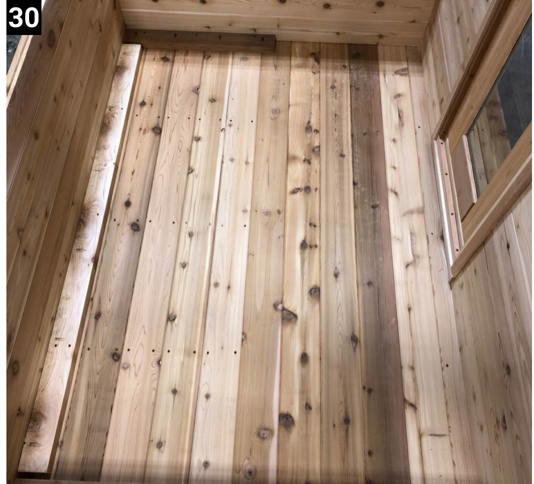
The Inside should look like this
