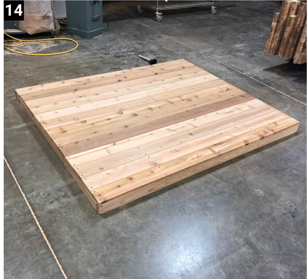
Completed floor should look like this. After the floor is completed the rest of assembly will need two people.
