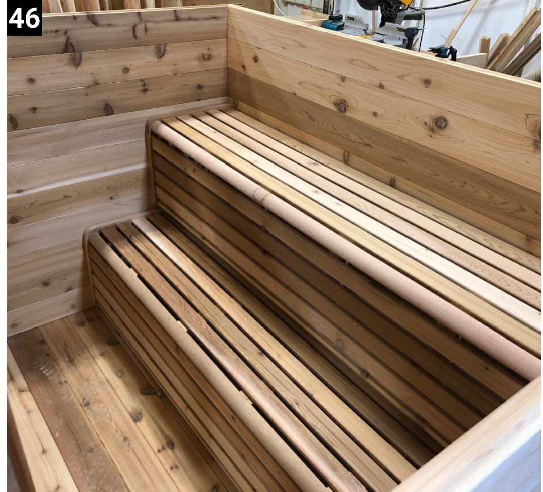
The inside of the sauna should look like this at this point
