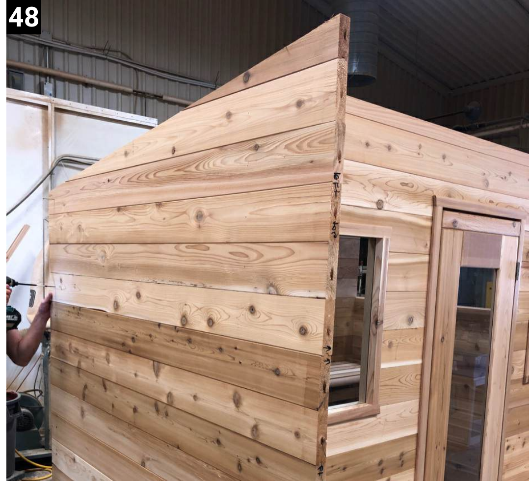
48 Put on both top side pieces. Screw them together with 4" screws and to the wall with 3" screws.
