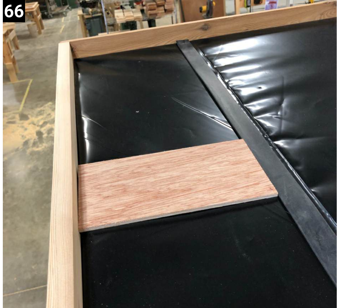
66 Staple or secure the neoprene strips to the roof, use the plywood spacer to properly space it from the side
