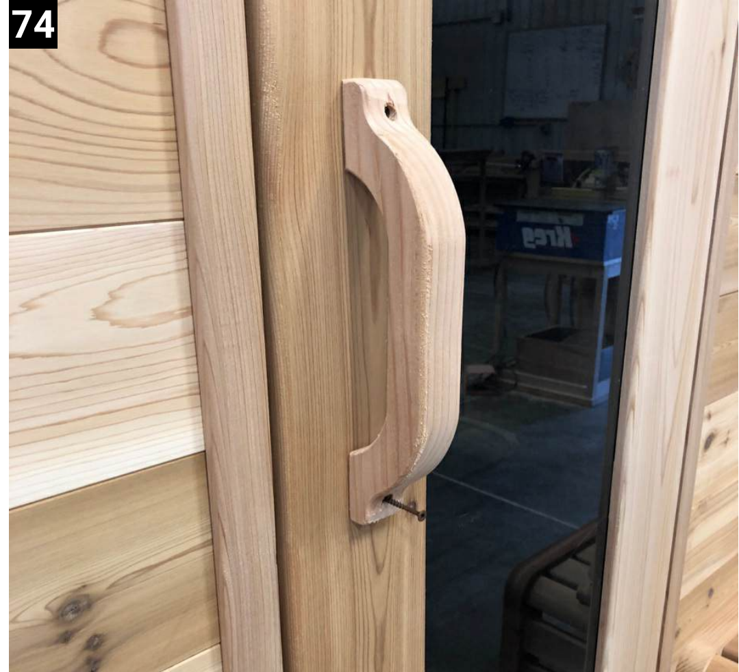
Put the small door handle on the outside of the door. Use 1 3/4" screws to secure it 25" down from the top of the door
