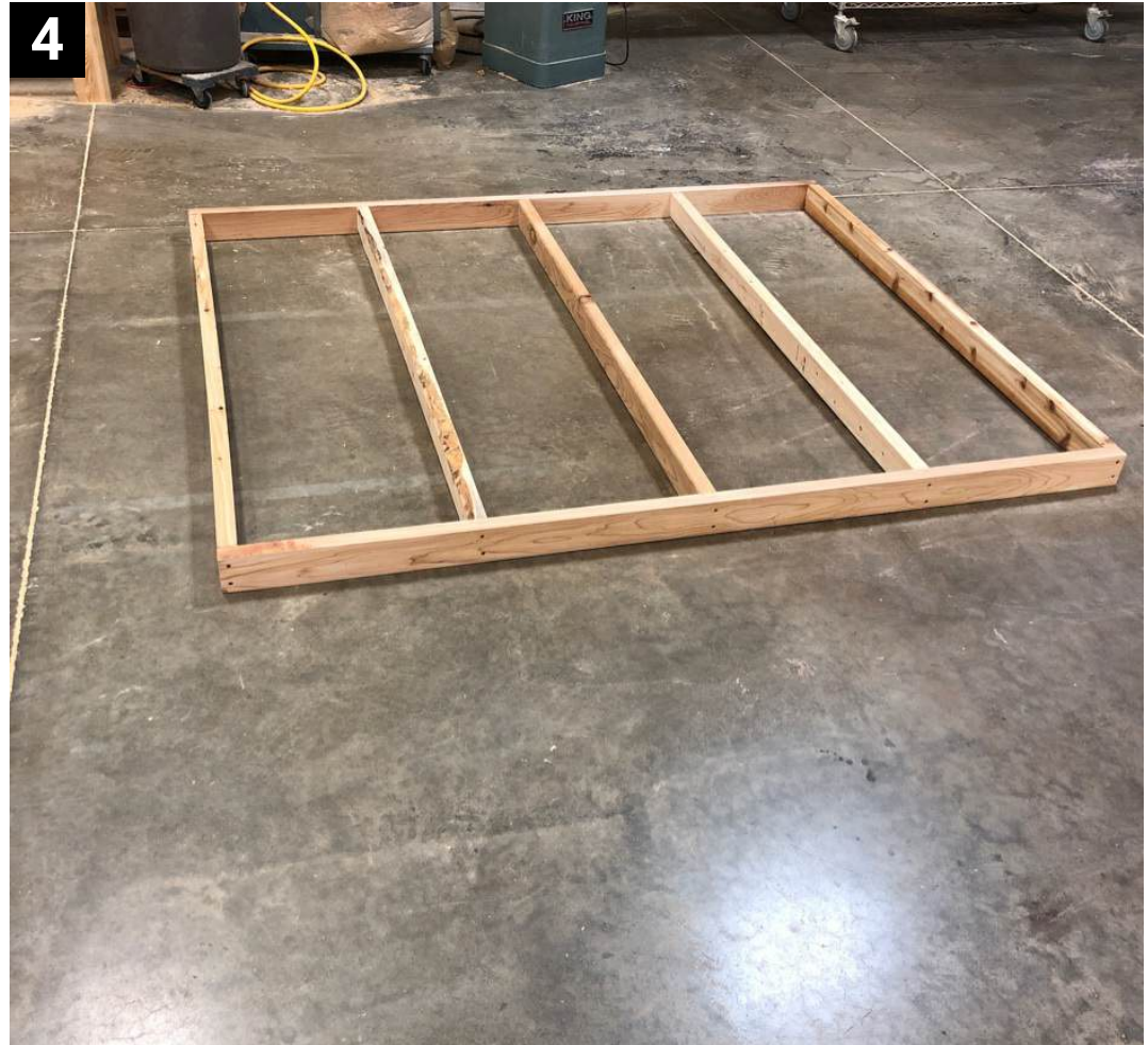
Finished floor frame should look like this.
