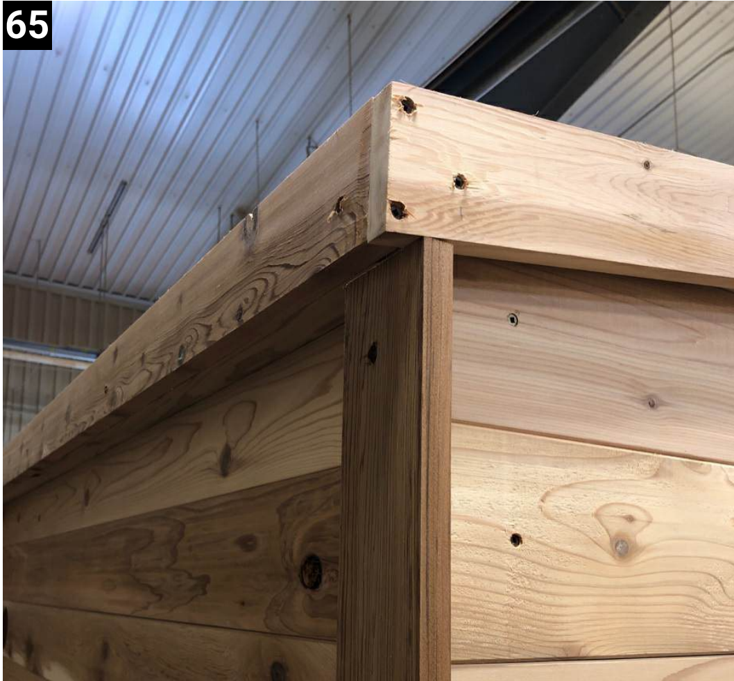
65 For the back barge boards, line up flush with the side barge boards.
