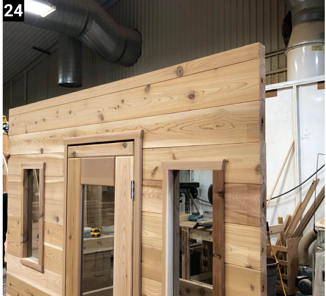
Slot the top piece of the front wall to complete the front wall.
