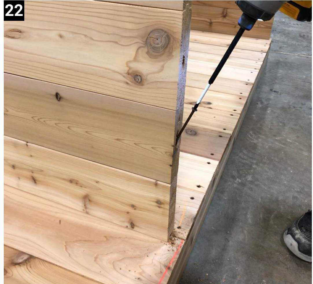
22 Using 4" screws and using the existing holes, attach the other side of the front wall together.
