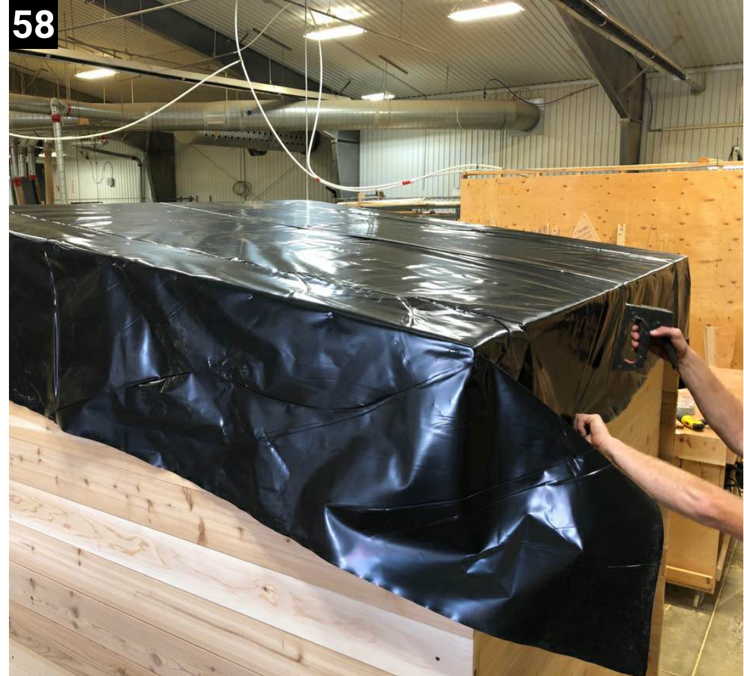
Drape roof membrane over and Staple to all the edges of the roof
