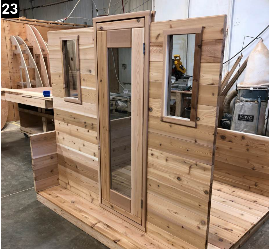
Sauna should look like this at this point
