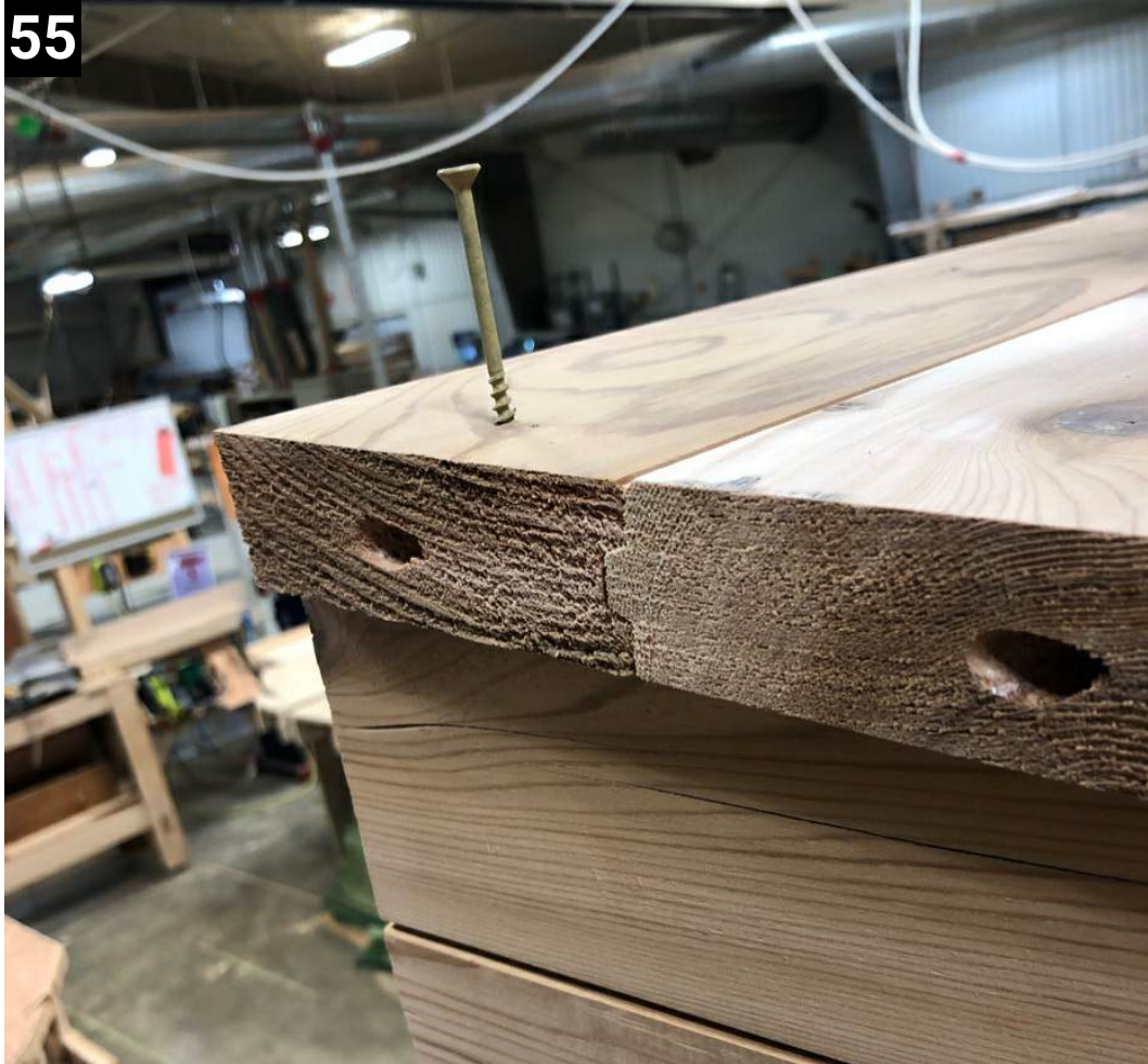
55 Center the roof on the body of the sauna and secure down with 3" screws
