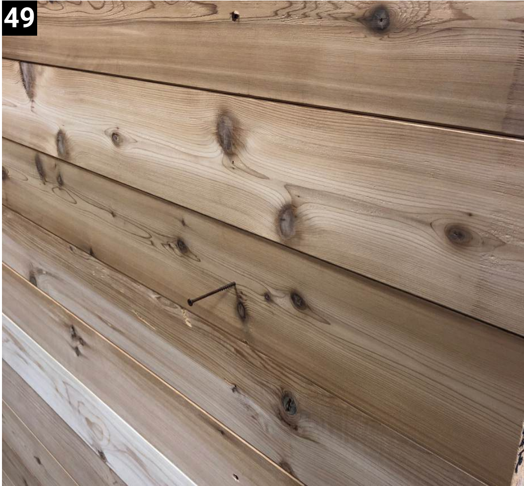
Screw 3" screws into all remaining pilot holes on the side walls.
