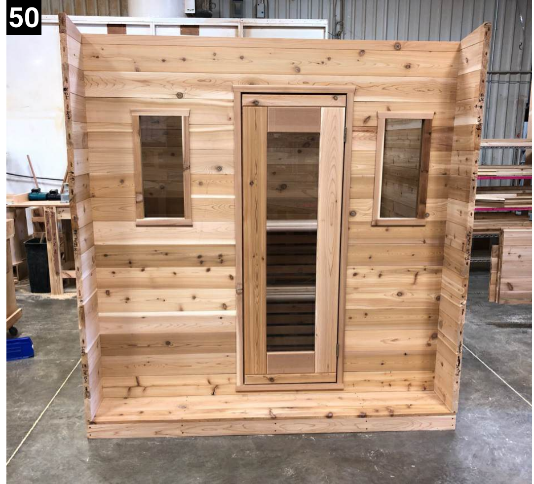
Sauna should look like this before installing the roof.
