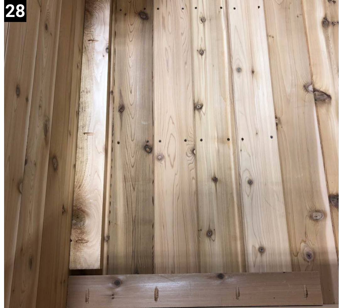
Place the three floor cleats as shown in the picture. Attach the back floor cleat to both the floor and the wall using 3" screws. Remember to only secure the back cleat at this time; do not attach the side cleats yet.
