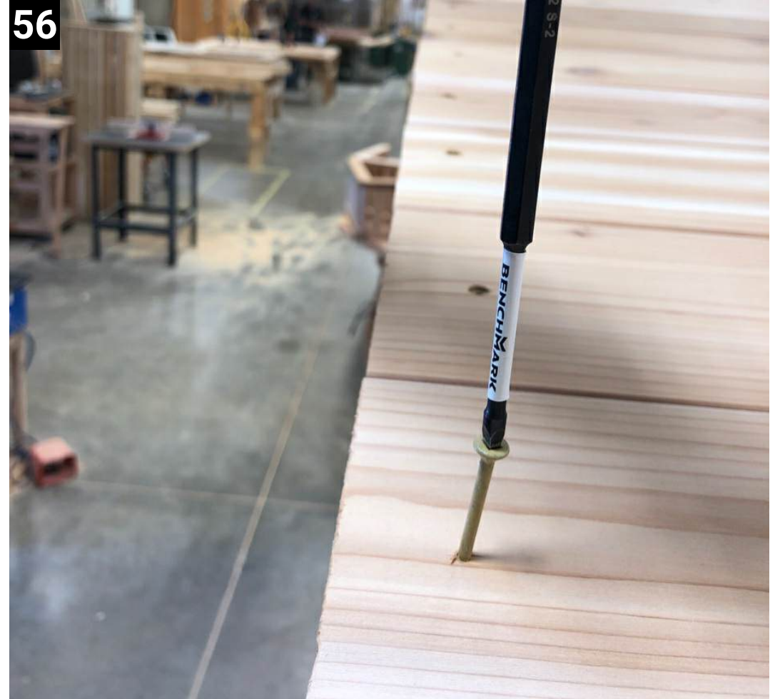
56 Sink a 3" screw in each end of every roof board.
