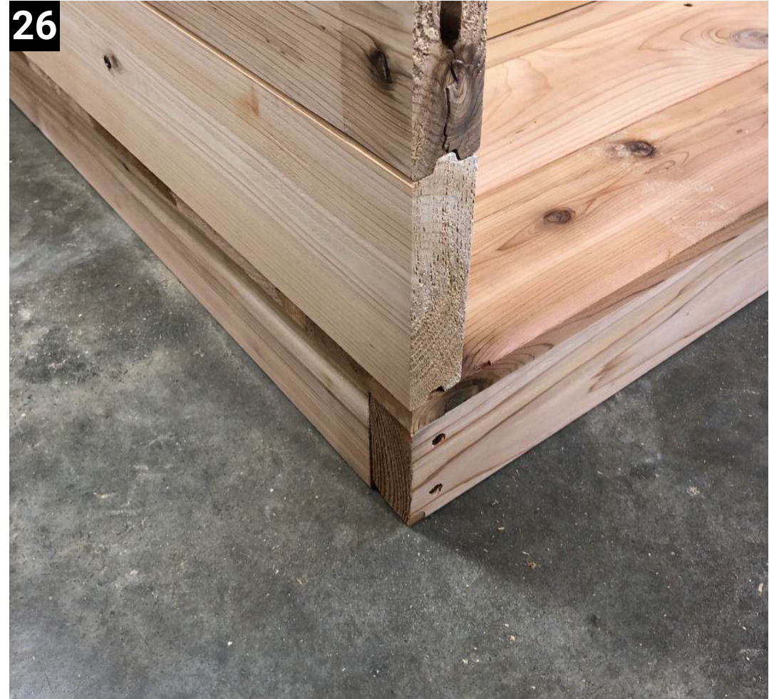
Make sure the front of the walls is even with the front of the floor frame, and place the sauna in the middle of the floor.
