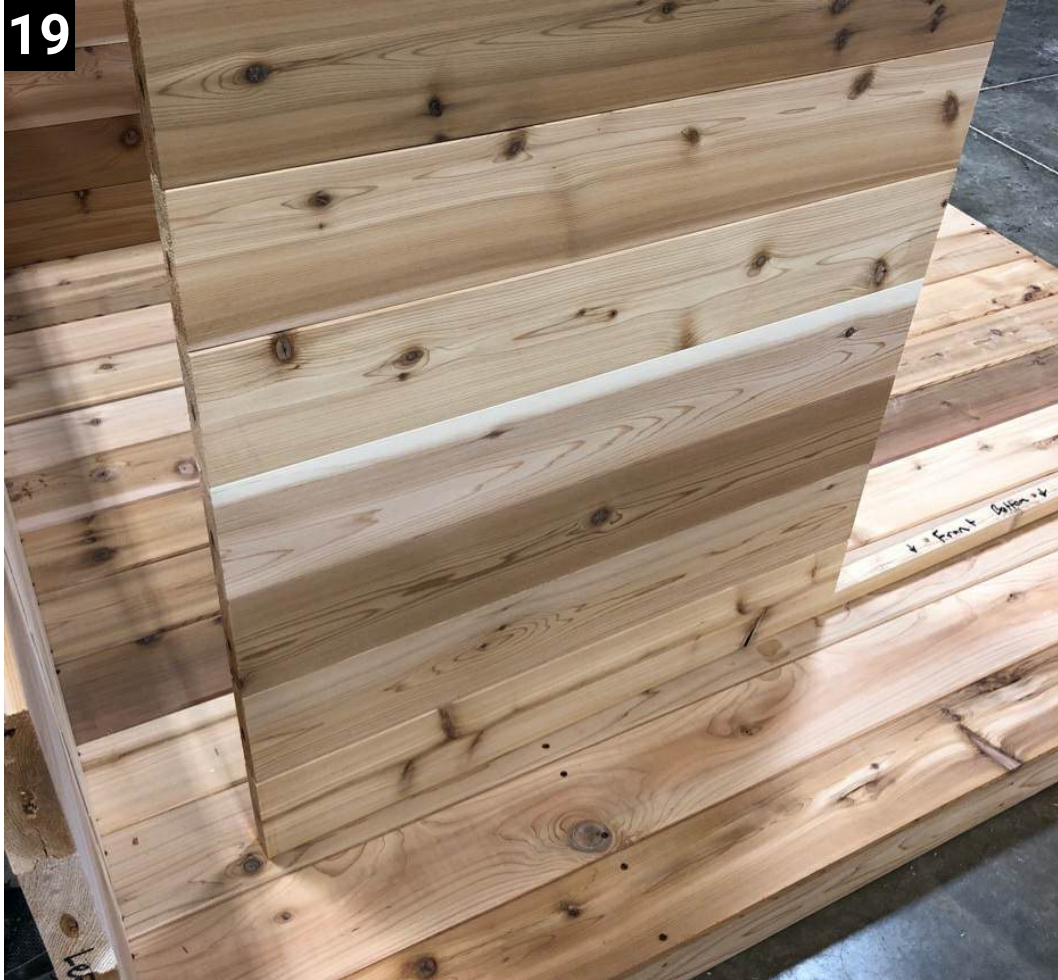
19 Connect one side of the front wall to the bottom part of the front wall.
