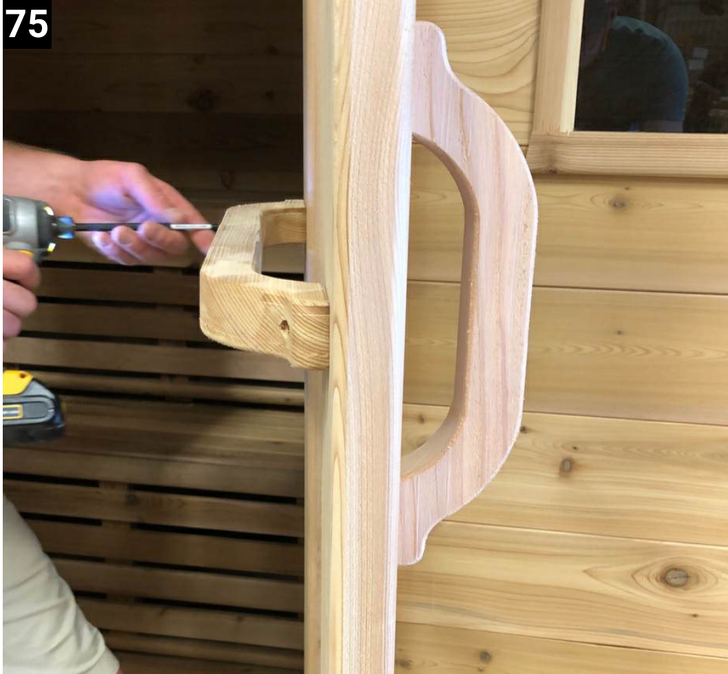
Put the large door handle horizontal across the door centered on the small door handle
