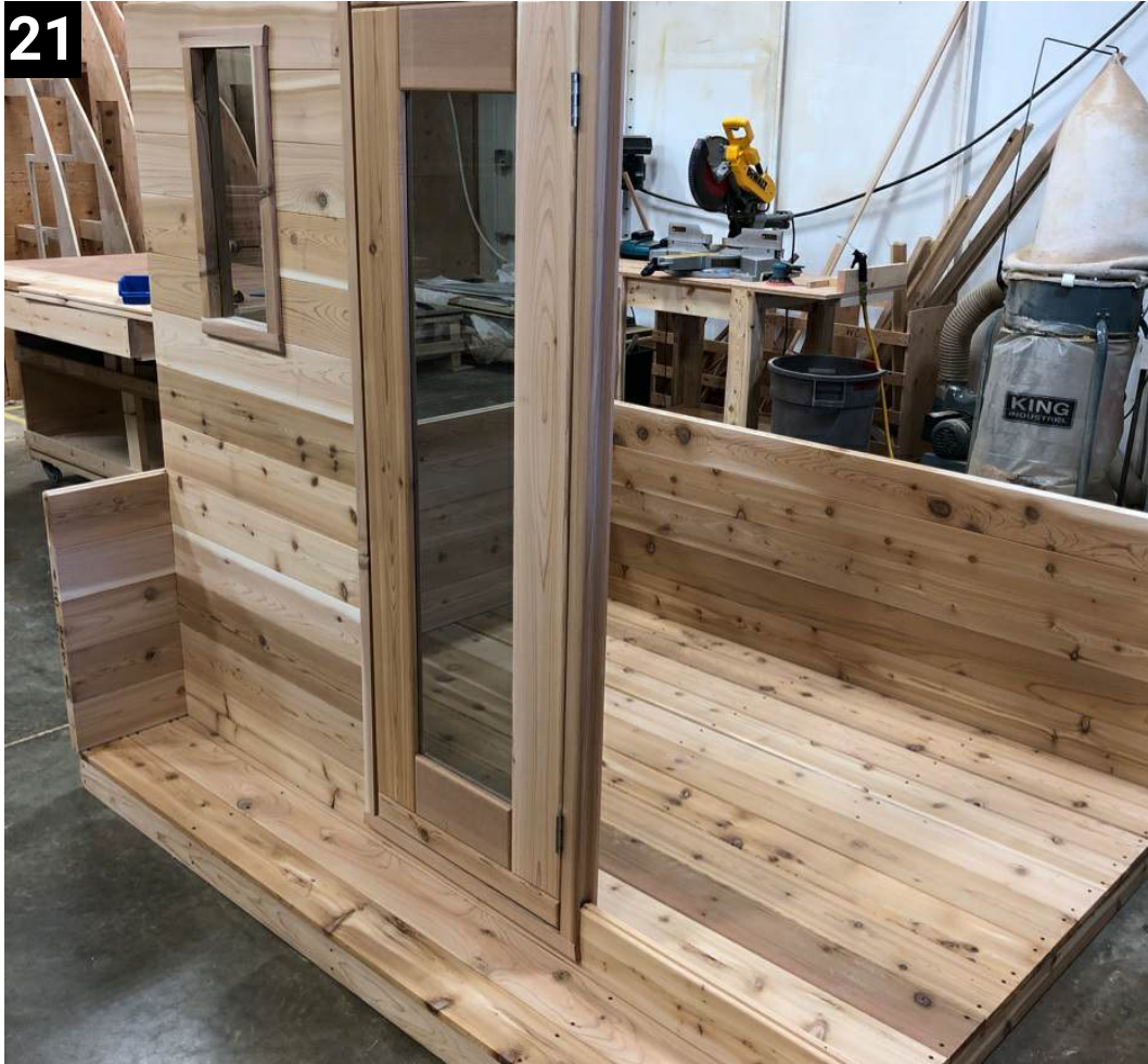
21 Slot the door into the front wall.
