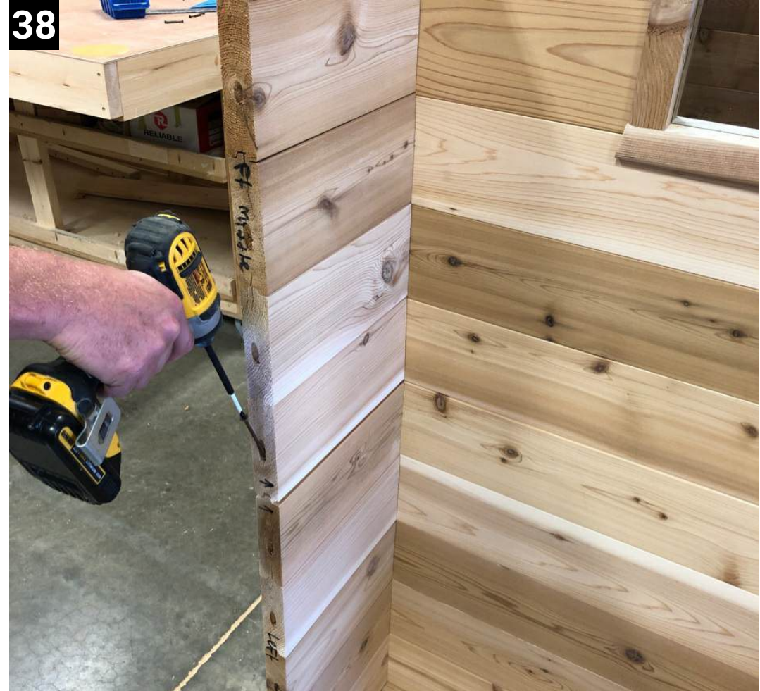
38 Slot the middle of each side wall in and attach to the bottom with 4" screws
