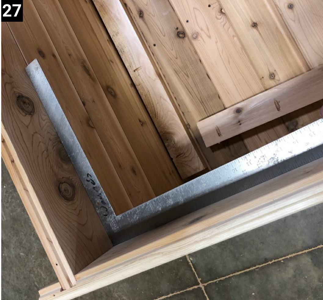
Check the inside of the sauna for square
