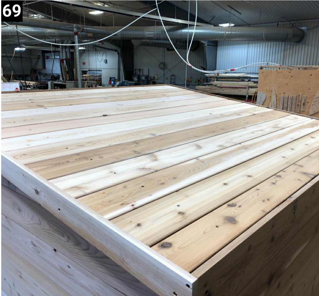
The roof should look like this when finished
