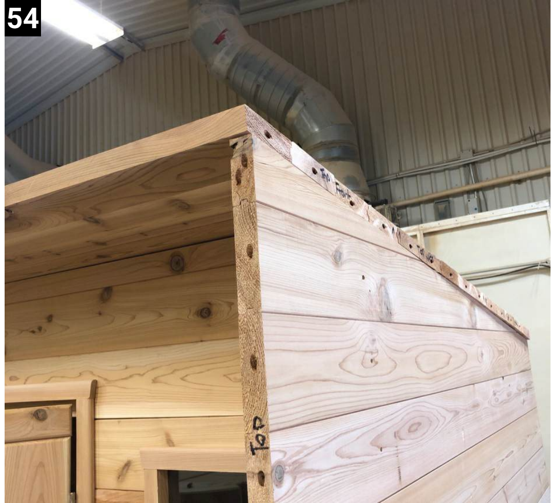
54 Place the top front piece on, and screw to the top middle piece with 4" screws. Make sure arrows are pointing up
