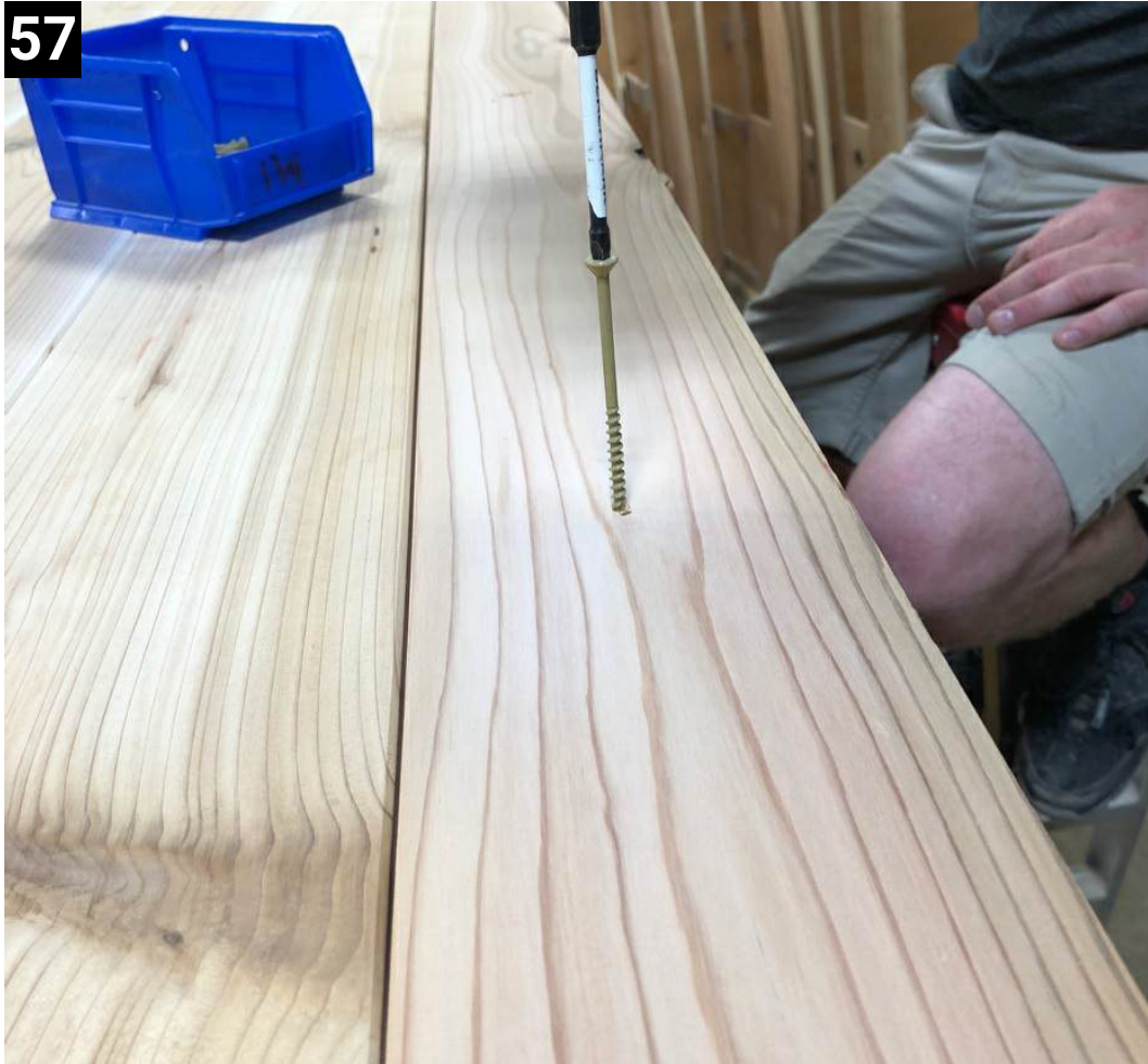
Secure the roof to the front and back wall with three 3" screws in each
