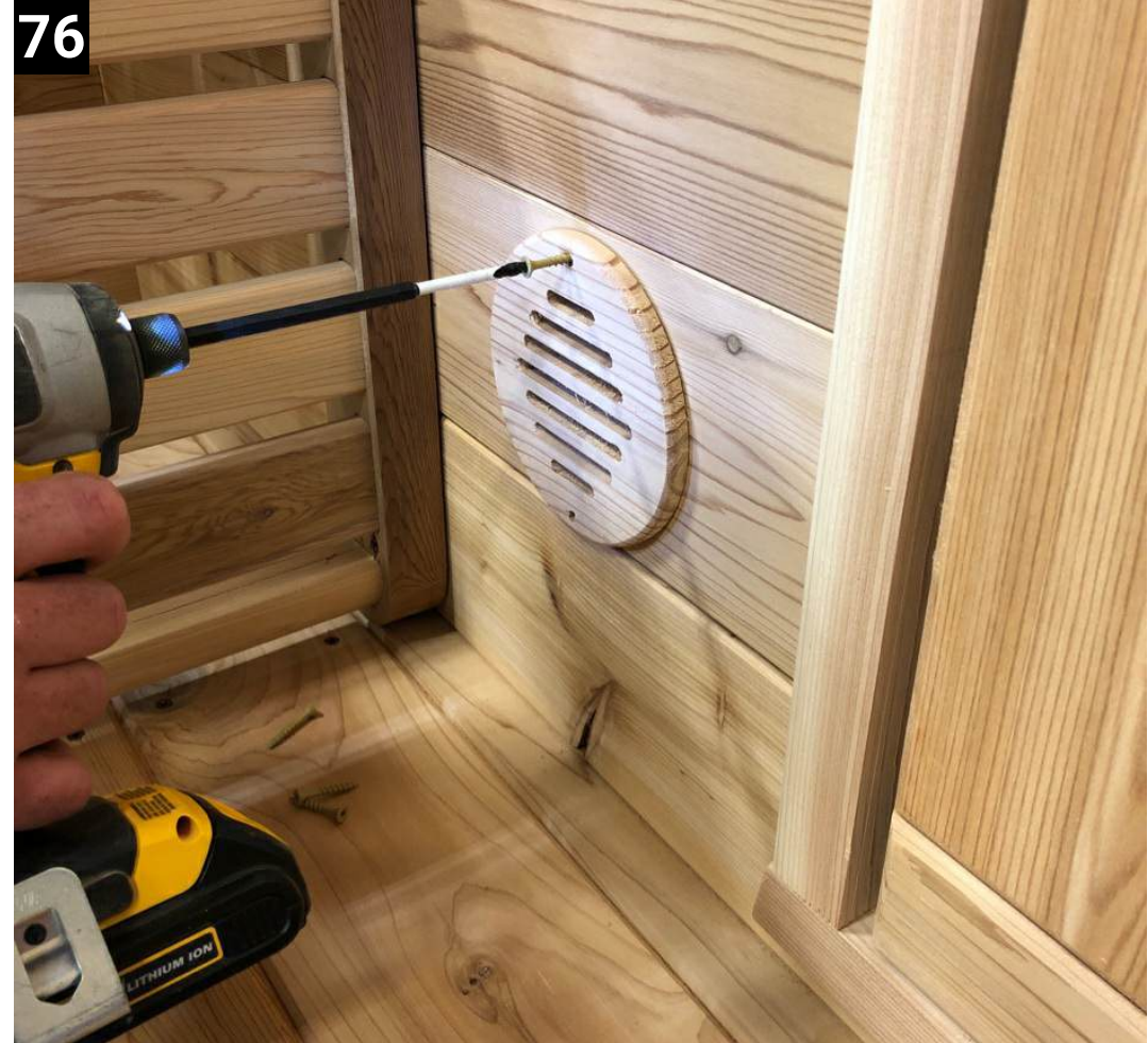
Put vents into the outside holes. Use 1 1/4" screws
