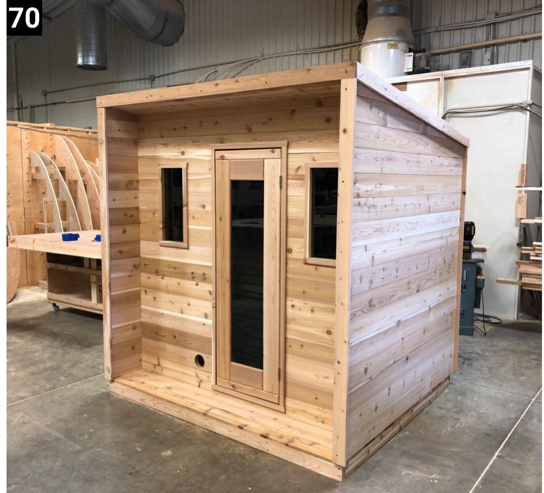
The sauna should look like this at this point of the build
