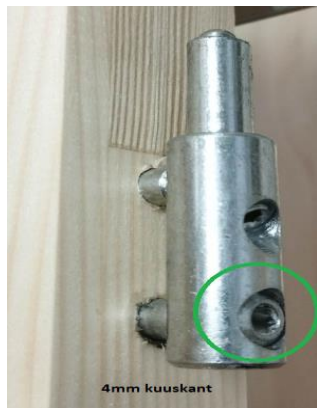
Fig.3 Door sash depth adjustment bolt
