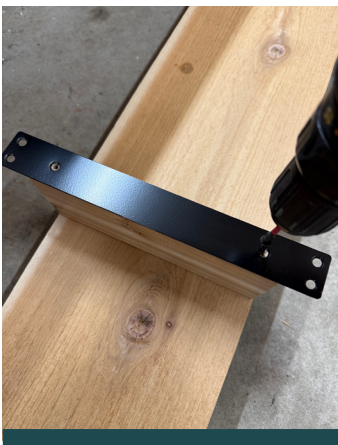
1. Attach mounting brackets.
