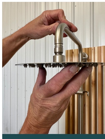
2. Thread shower head onto stem and gently tighten with wrench.
