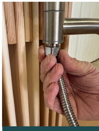
3. Thread hose onto valve assembly as shown and gently tighten with wrench.
